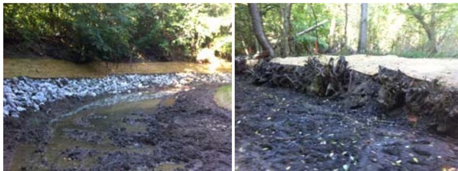
Photos of work (left to right): rock toe with erosion control mat above; root wads (tree trunks into the eroded shoreline)
