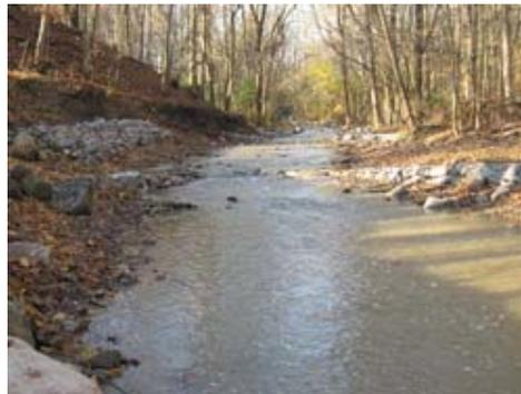
Erosion and downcutting in the State Road Drain were addressed using innovative techniques including cross vanes, riffles and pools, pictured here. This photo was taken in Nov., 2012.
