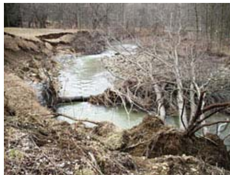
Streambank slope before construction
