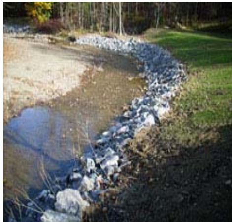
Streambank slope after construction
