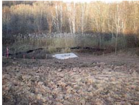
Embankment after construction
