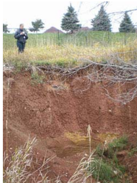
Embankment before construction
