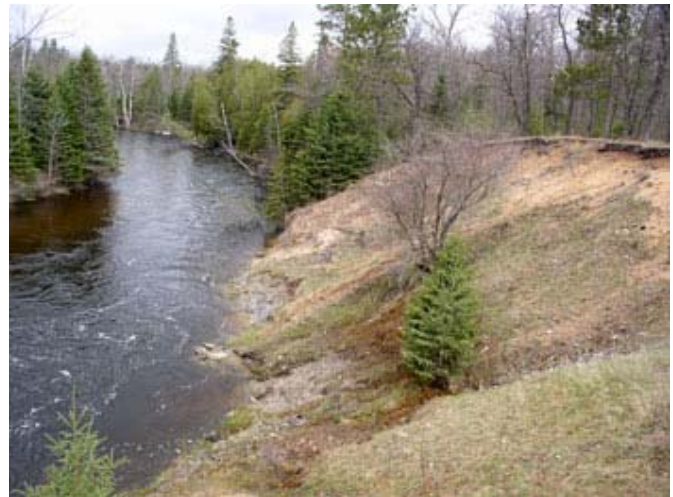
Photo: Black River 2006, prior to any erosion control work Project #15: Upper Black River Bio-Erosion Control Grantee: Huron Pines, MI
